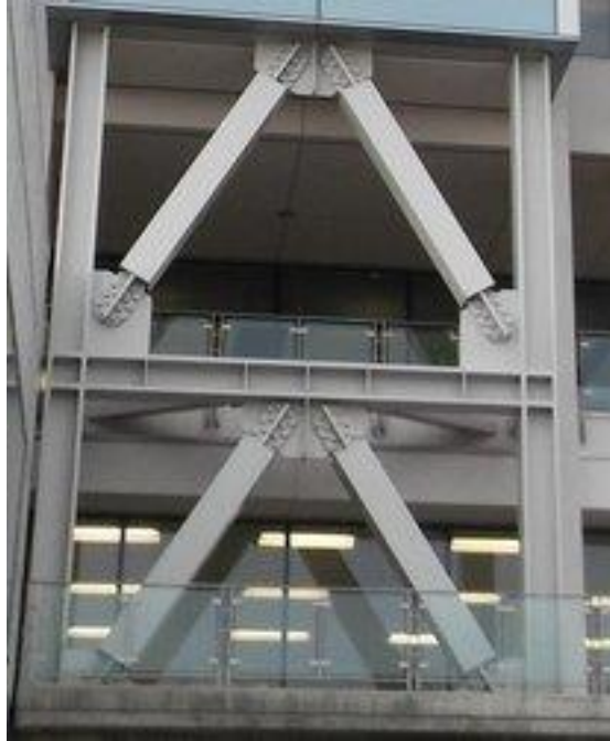
Figure 1.1 BRBs applied in the J. William Marriott Library at the University of Utah
