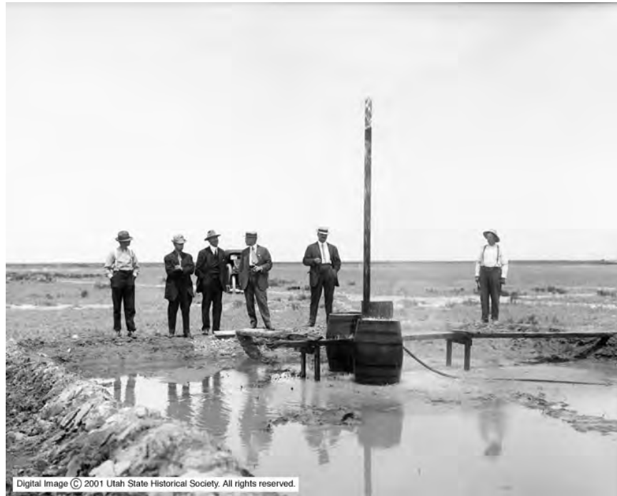
Figure 3 - Highland Improvement Company Well (1914)
