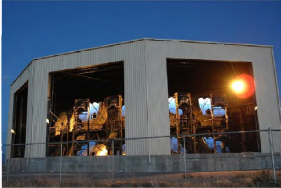
Figure 1.11: Picture of Black Rock Mesa (BRM) FD building with the telescope doors open showing the segmented focusing mirrors.
