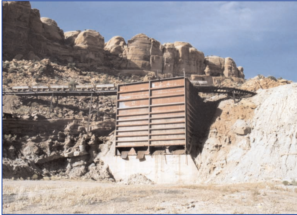
Ore bins and hauling area for the Mi Vida mine, Lisbon valley mining district.
