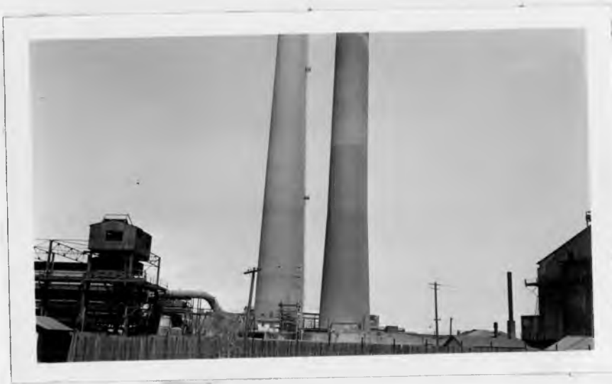
Partial view of American Smelting and Refining Plant Murray, Utah.
