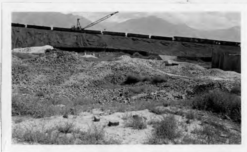
Slag Dump of the American Smelting and Refining Company (west side view)
