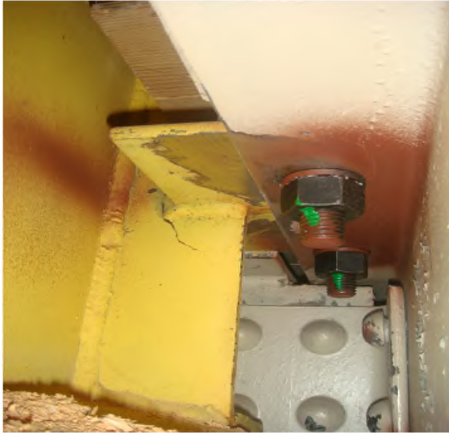
Figure 38 Fatigue crack found visually at Point Barrow, Alaska in July 2011
