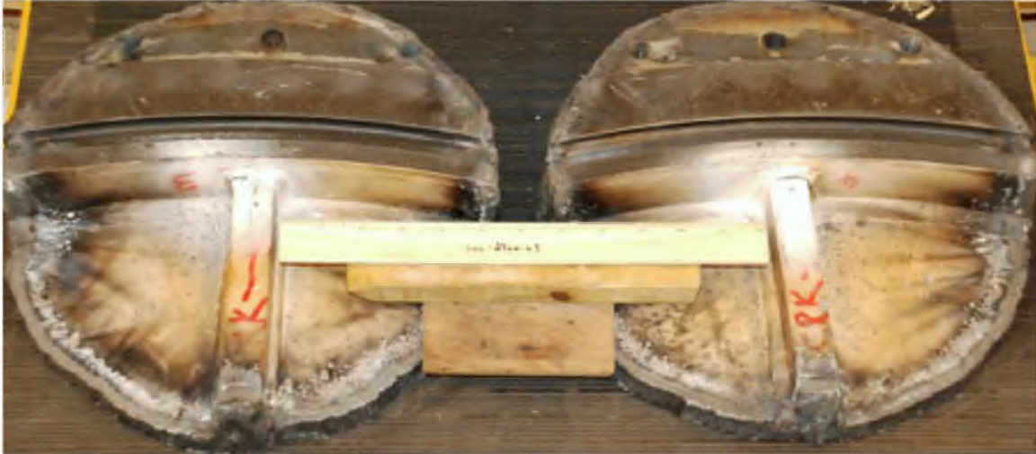
Figure 45 Bearing support sections containing cracks 3 & 4 at ends of the spokes
