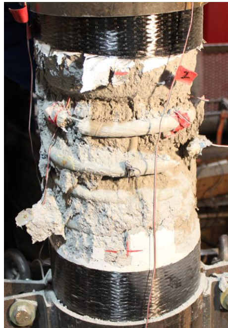
Figure 3.8: Concrete prism reinforced with GFRP spiral #5@2.5 at failure.
