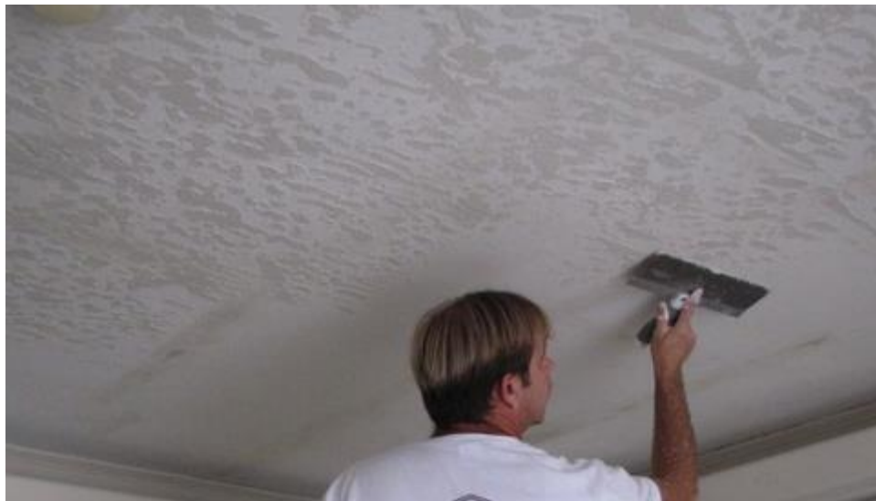
Figure 7. Worker applying drywall texture. Adapted from “Skip-Trowel Texture,” by K. B. Marks, n.d. Retrieved from http://www.paintandart.net/Skip-trowel-texture.jpg . Copyright n.d., by Bill Marks Painting.
