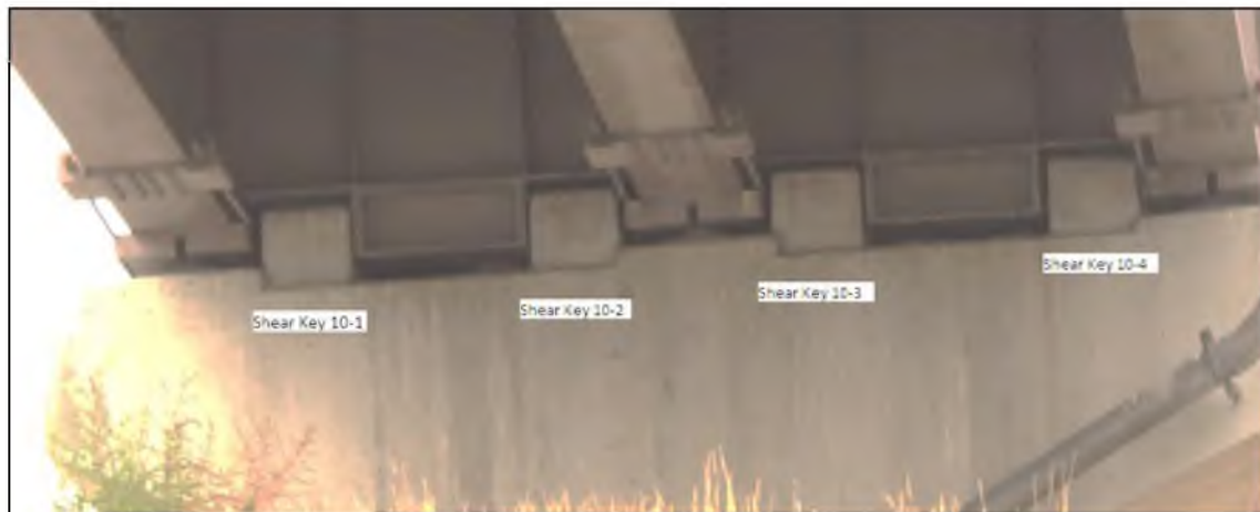
Figure 4.18 Shear keys on the bridge bent
