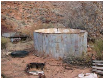
005- steel water tank
