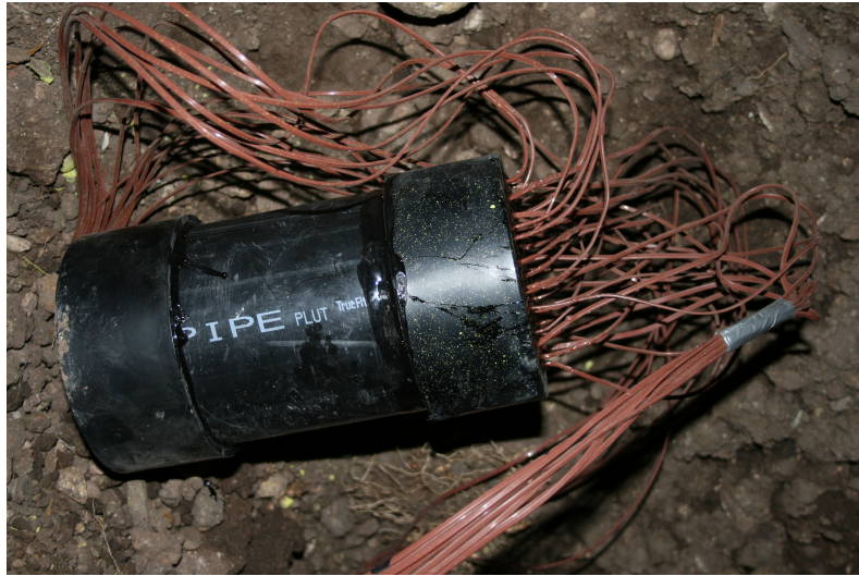
Figure 2.17: Thermocouple Enclosure: Final Product. The finished thermocouple junction enclosure.
