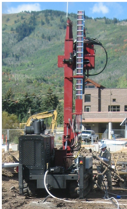
Figure 2.28: The Borehole Drilling Rig: View 1
