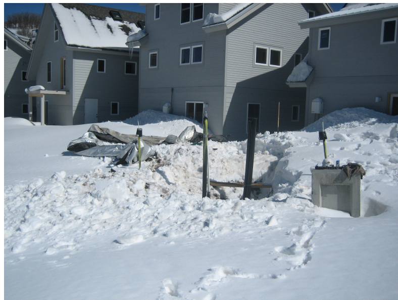
Figure 2.36: Snow During Construction. Weather drastically slowed the pace of construction.
