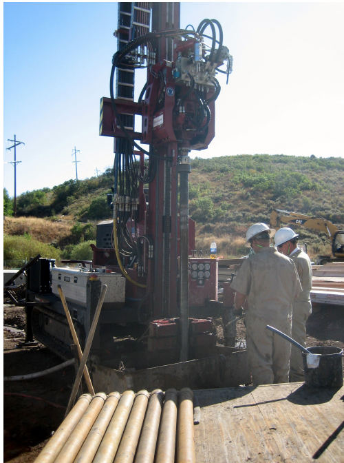
Figure 2.29: The Borehole Drilling Rig: View 2
