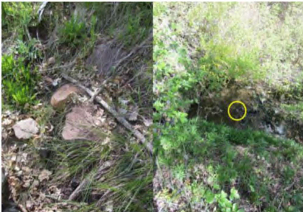
Figure 3.11. Rockfall adjacent to Slope # 2, pane on left shows angular boulders covered in soil and vegetation, pane of the right shows a more recent fall with a boulder in Parleys Fork (5/10/2012)
