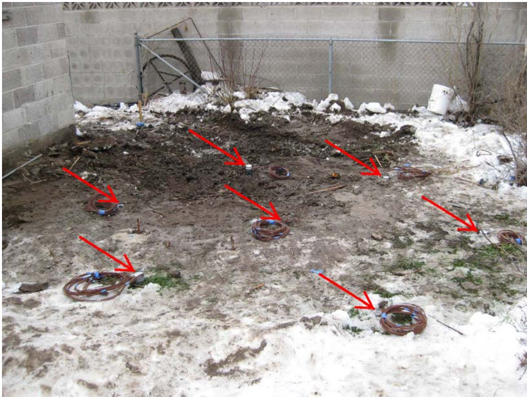
Figure 4.3. Thermosiphon pipes installed. Pipe locations indicated with red arrows.
