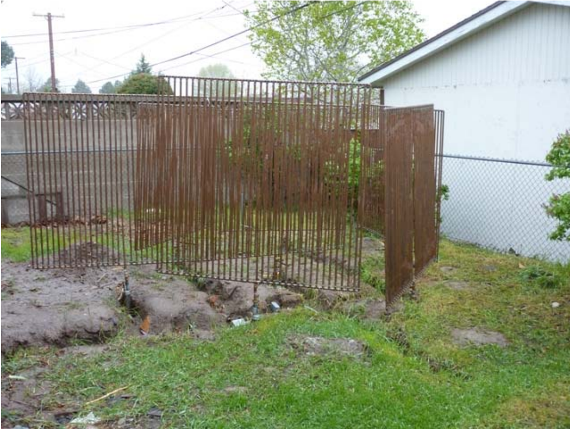
Figure 4.4. Thermosiphons with heat exchangers.
