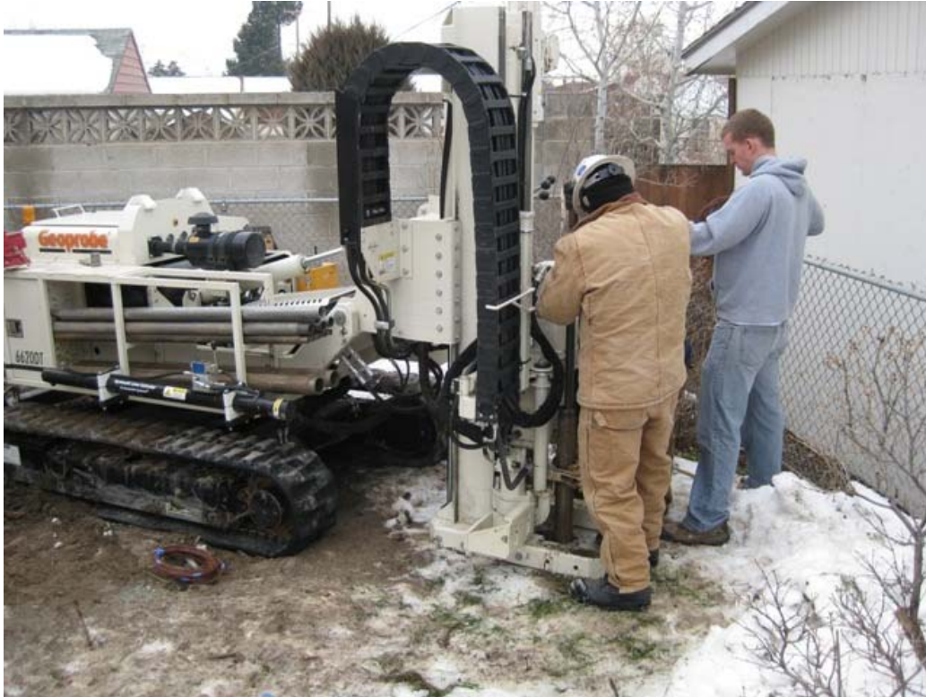
Figure 4.2. Direct-push drilling, using a pneumatic hammer and expendable tip.
