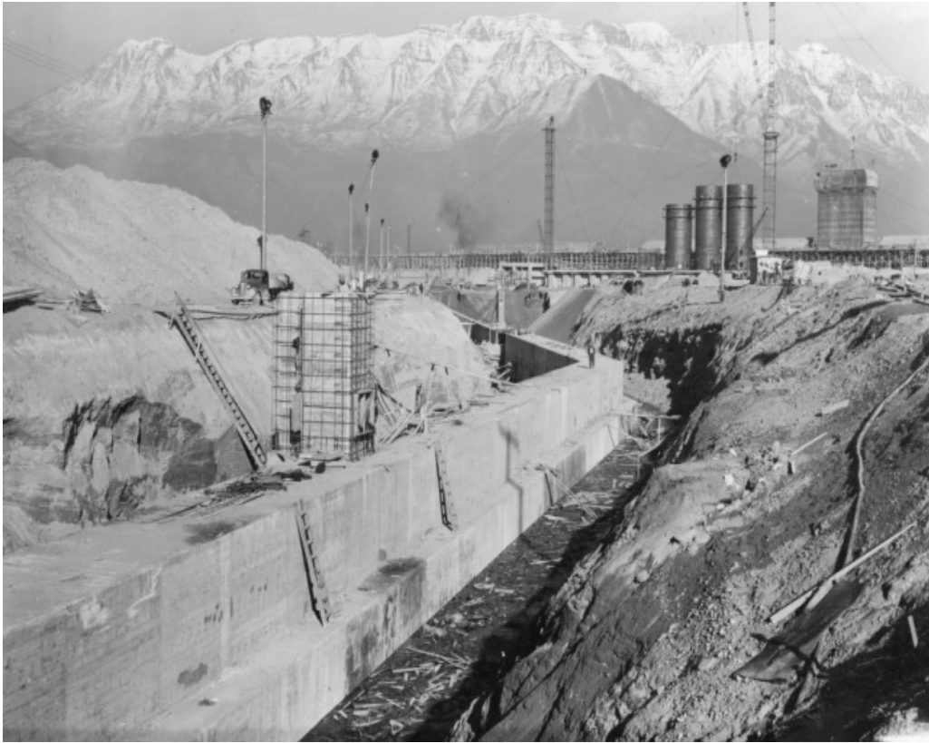
Figure 2: Water Tunnel Under Construction at the Geneva plant, November 1942
