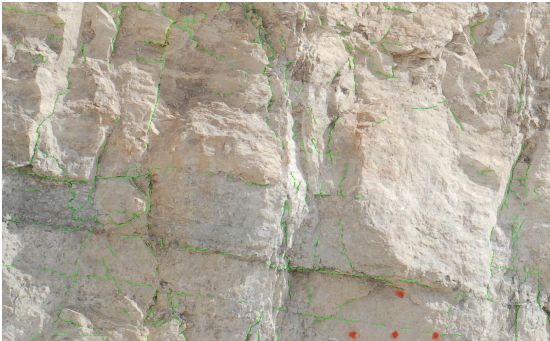
Figure 37: Manual delineation of existing rock joints
