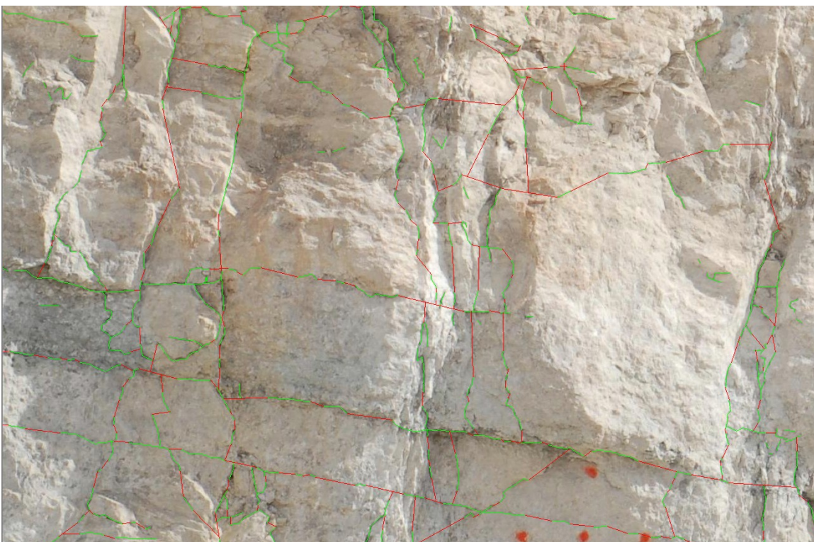
Figure 54: Traces in Limestone Overburden. Joints in green, bridges in red.
