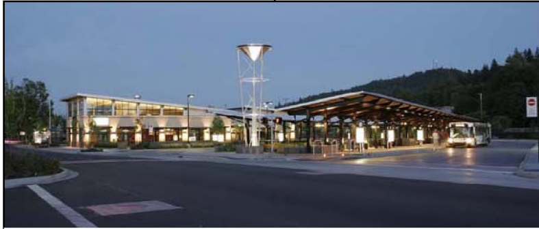
Springfield Station was planned to become a community hub as well as an element that would focus high density development. Image courtesy of Jack Gonsalves.
