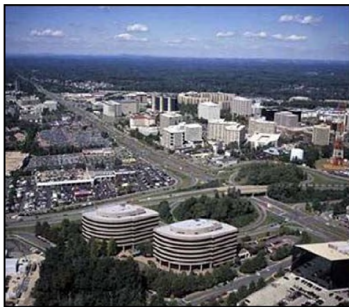
Tyson's Corner, located on the Dulles Metrorail Extension project.
