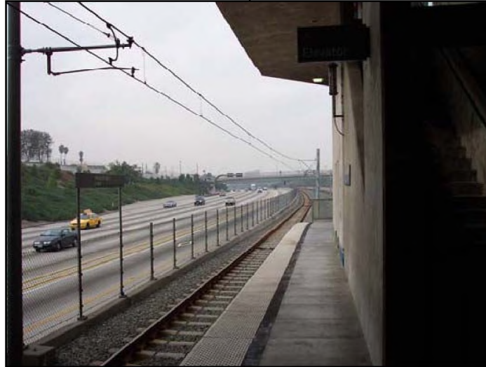
Los Angeles' Green Line is located in a highway right-of-way. Photo courtesy of Susan Herrc.
