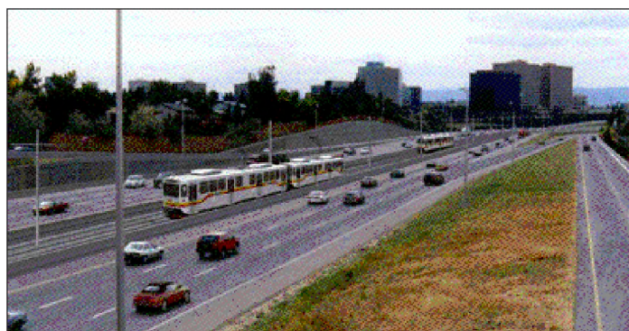
Denver's Southeast Corridor in the highway right-of-way. Photo courtesy of Tim Van Meter, Van Meter Williams Pollock.
