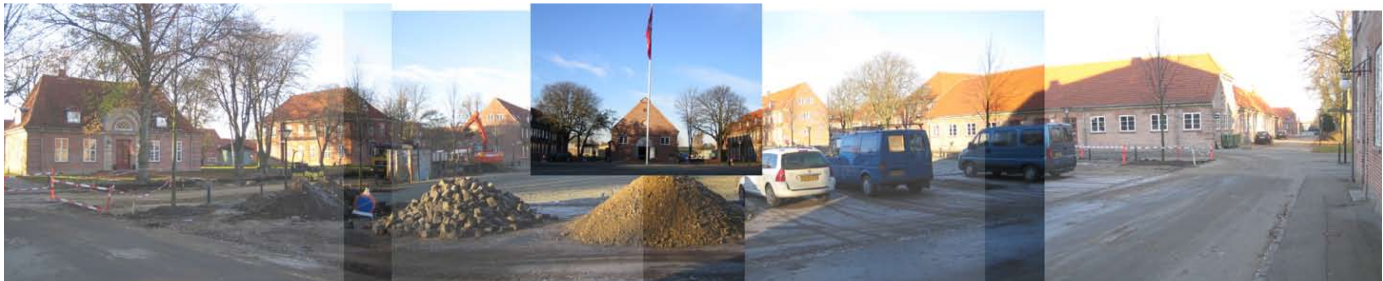
Site B. Panoramic View of Site
