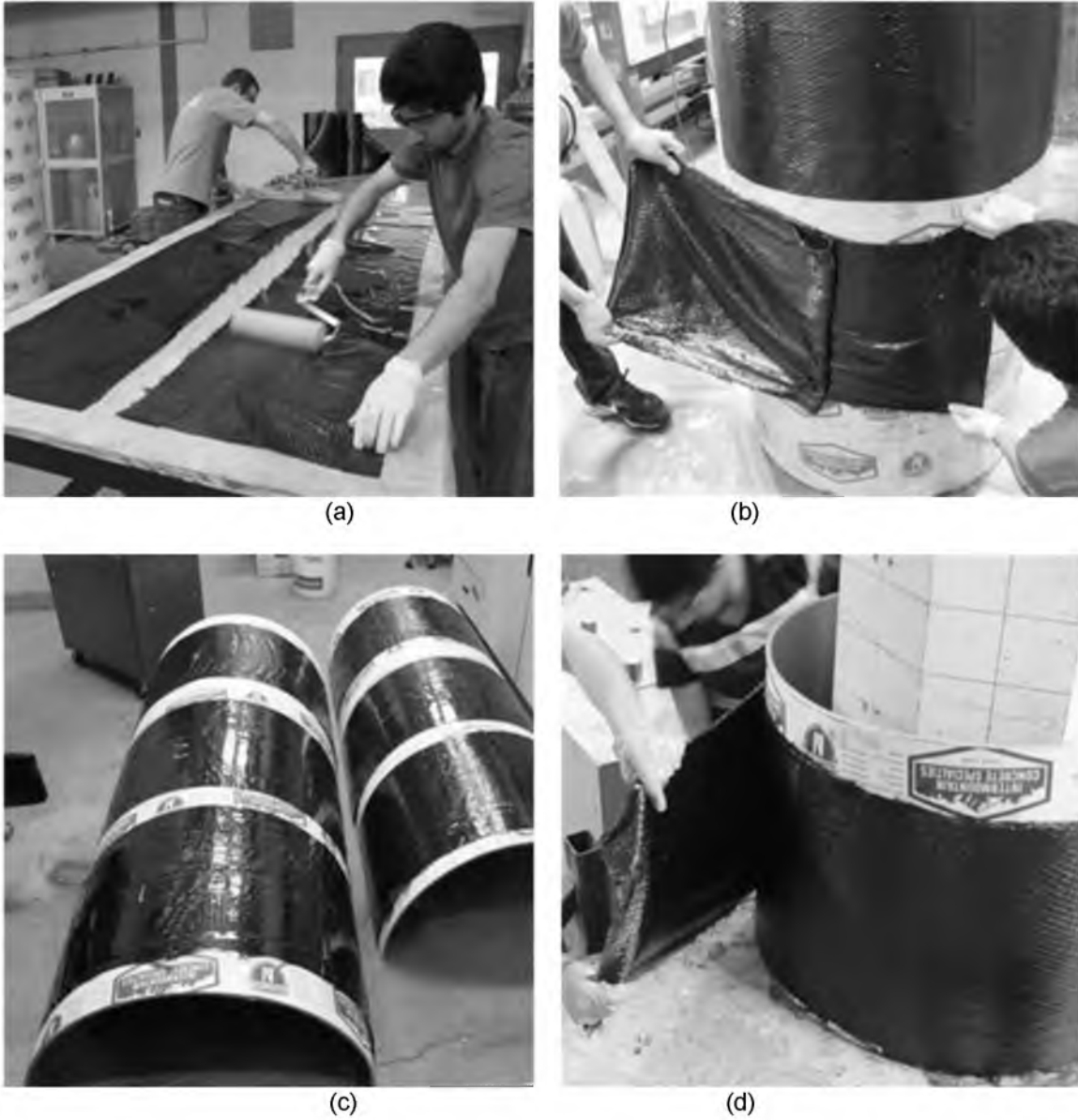
Figure 3.3 – CFRP preparation: (a) Saturation, (b) Making of prefabricated shells, (c) Prefabricated shells split into two, (d) Wet layup
