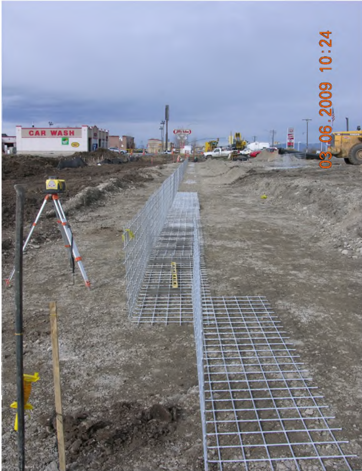
Figure 1-9. Welded wire mesh used for facing of MSE wall.
