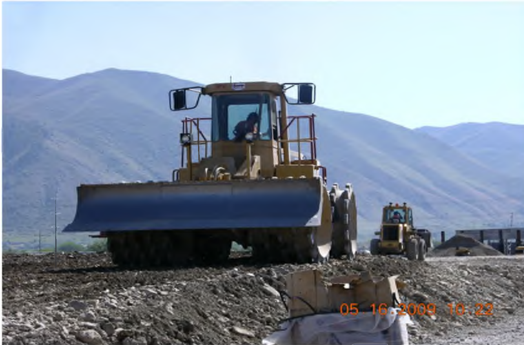
Figure 1-7. Compaction of fill.
