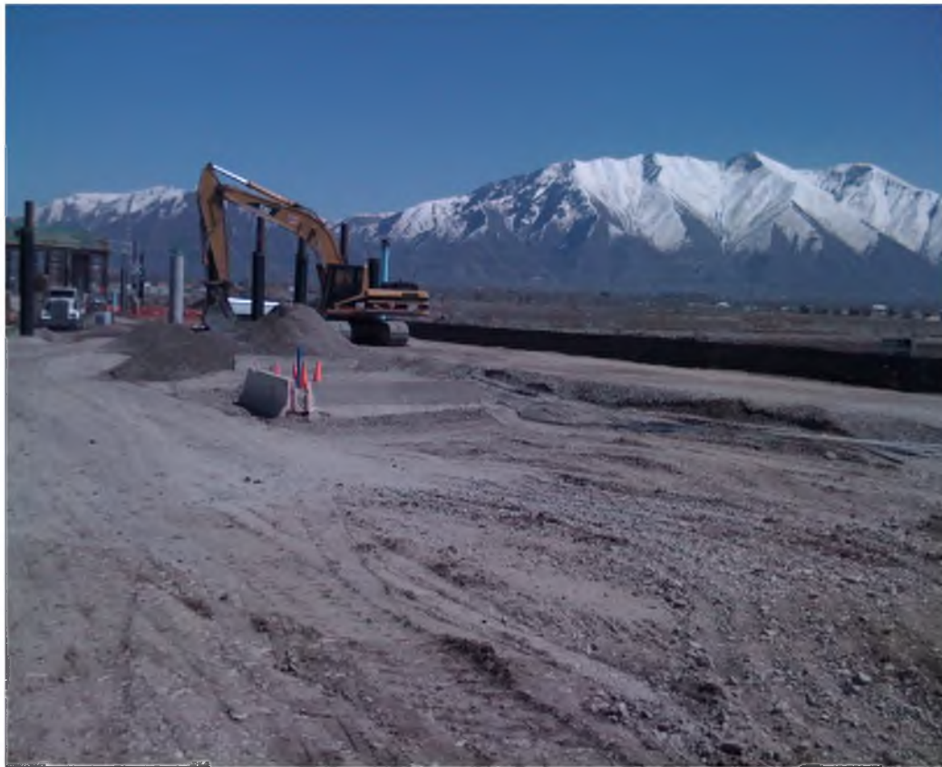
Figure 1-6. Initial fill height just after instrumentation was installed on April 20, 2009.
