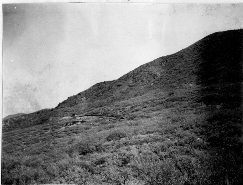
"Wasatch Tunnel from road."
