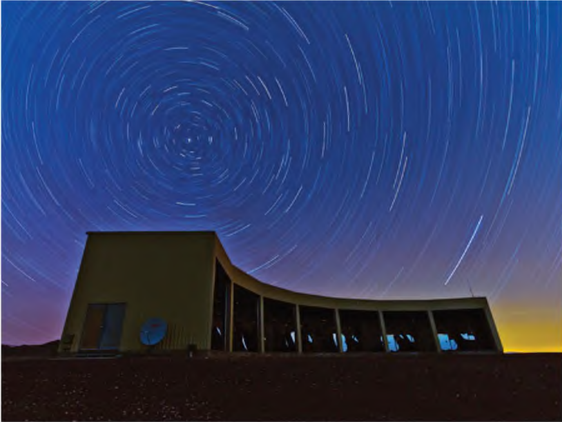
Figure 3.13. Middle Drum Fluorescence Detector (MDFD): 14 telescopes view the southern night sky 3^\circ to 31^\circ in elevation.
