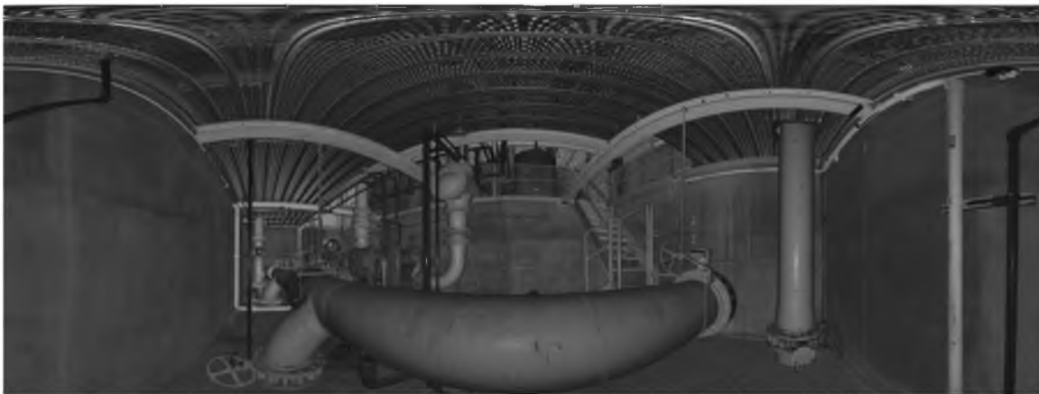
Figure 1-2 Measured brightness data acquired by a LiDAR scanner
