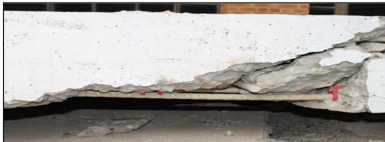
Fig. 2.8 Deformation of GFRP bars at bottom of panels after shear failure
